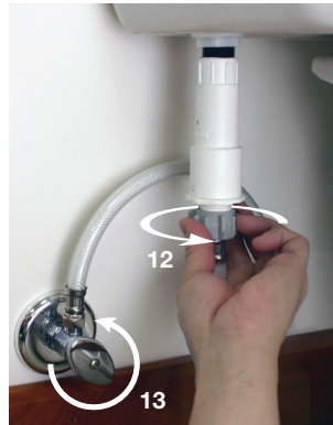
12. Connect supply line to EXTERNAL REGULATOR, hand tighten. 13. Rotate handle of water supply stop counter-clockwise to fully open the water supply.
