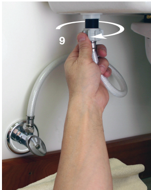
9. Disconnect the water supply line from the lower supply shank. Be prepared to collect a small amount of residual water from the supply line.
