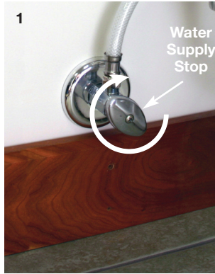
1. Rotate handle of water supply stop clockwise to turn off water.
